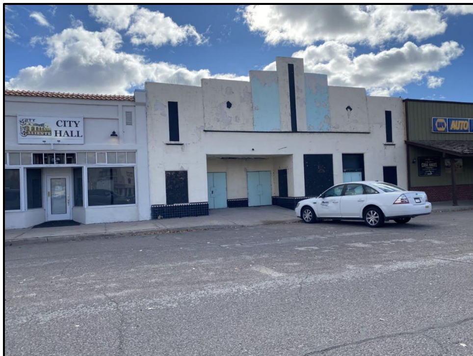
1. View looking southerly at the northern elevation.
