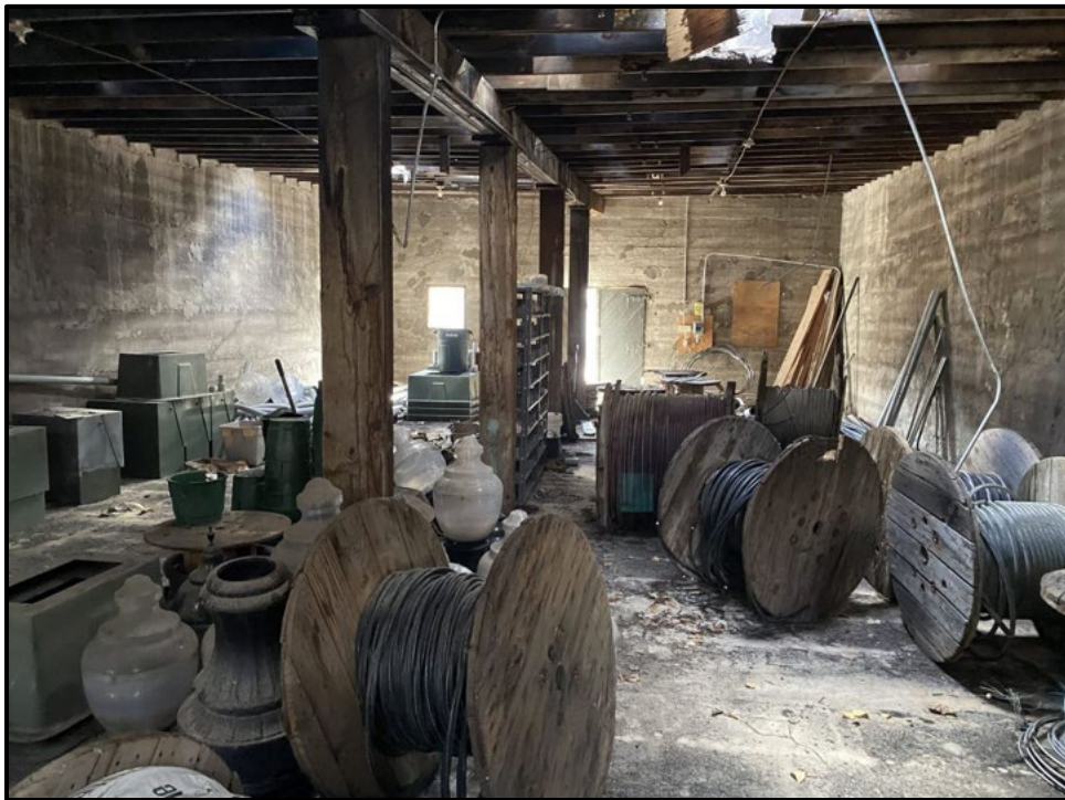
9. Additional interior view looking south.
