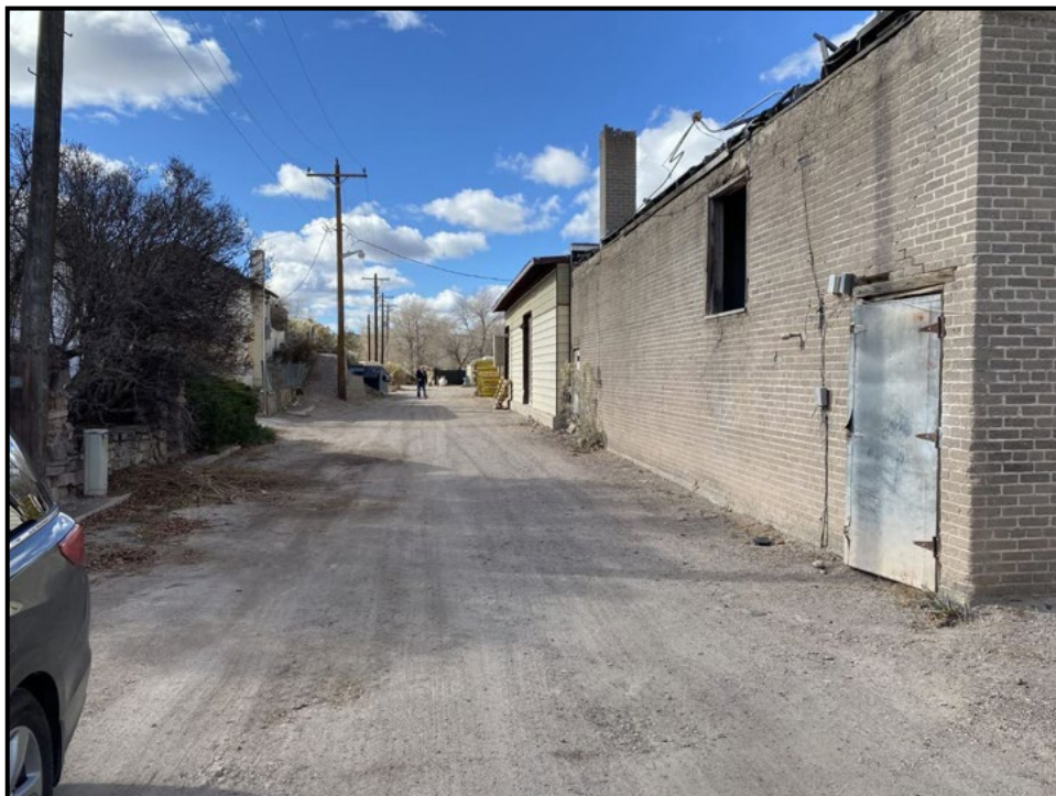
3. Street scene looking westerly along Clark Street. The subject can be seen in the right foreground.
