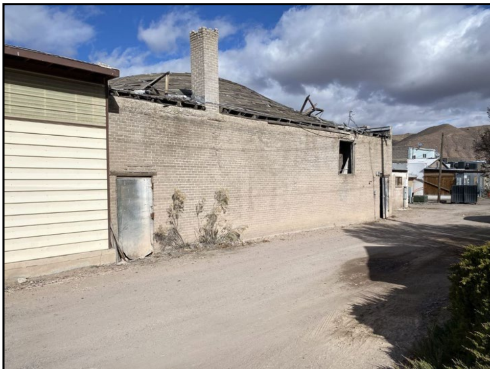
4. View looking northeasterly at the southern elevation.
