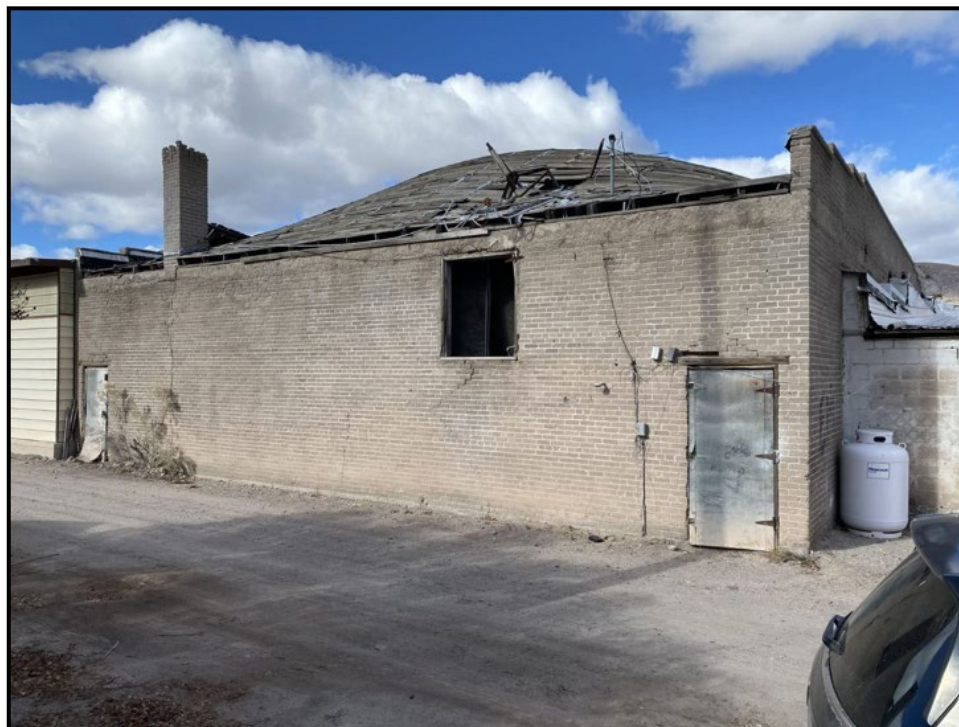
2. View looking northwesterly at the southern elevation.
