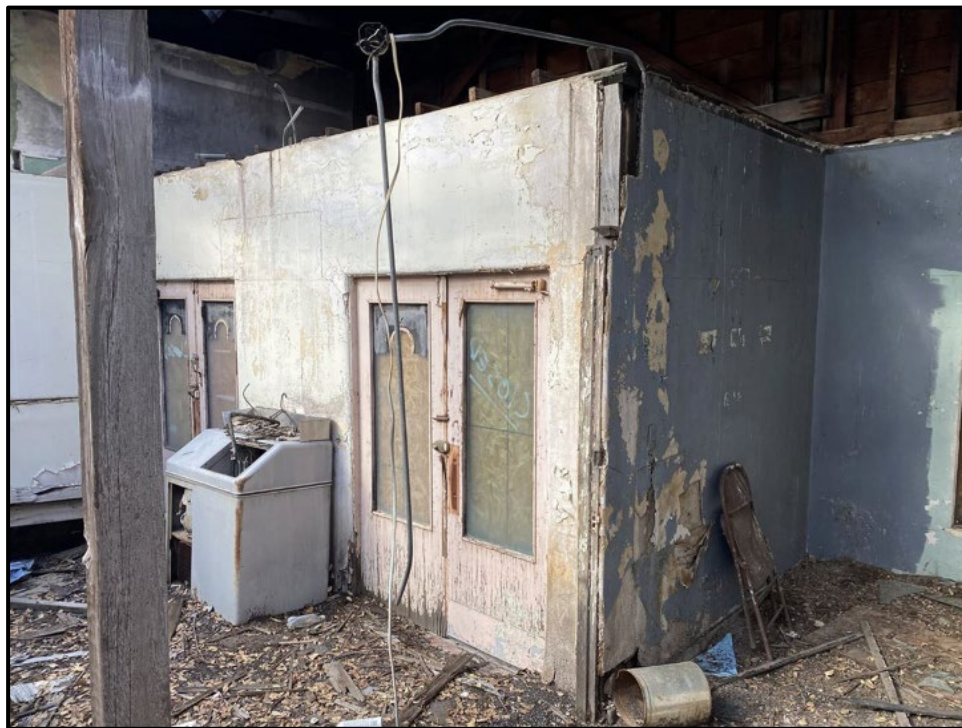
10. View of the front of the building, near the entrance.
