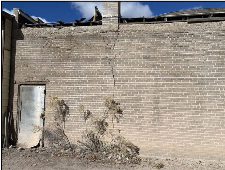
6. View looking northerly at a western portion of the southern elevation.
