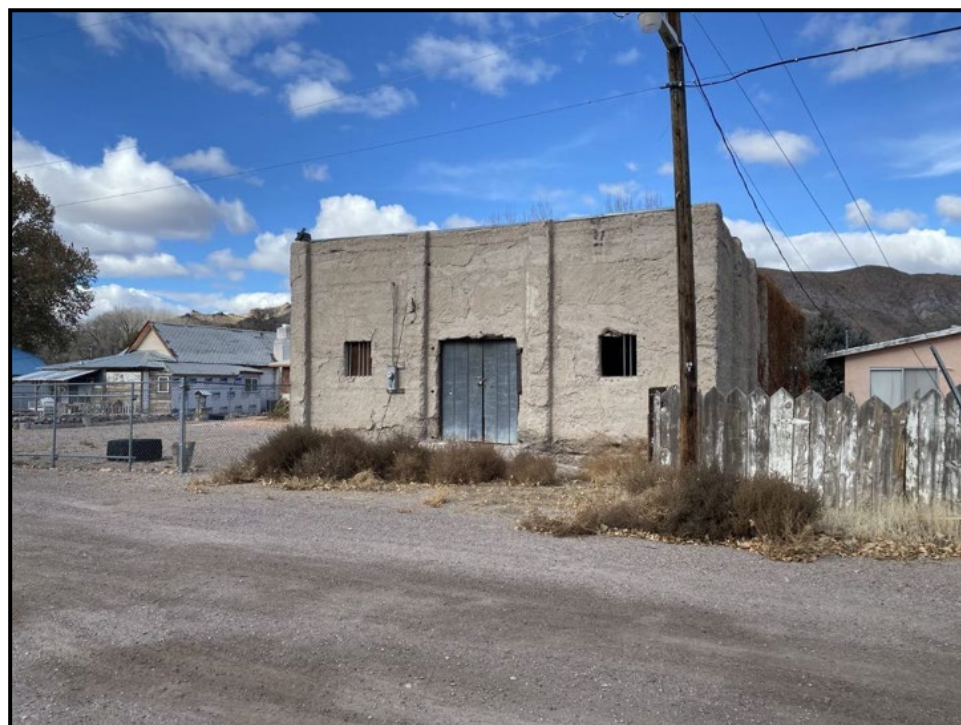
4. View looking northerly at the southern and eastern elevations.
