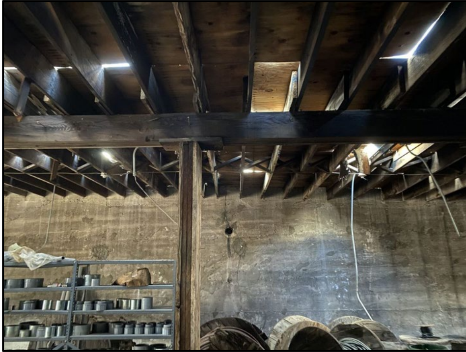
10. Interior view of the ceiling.
