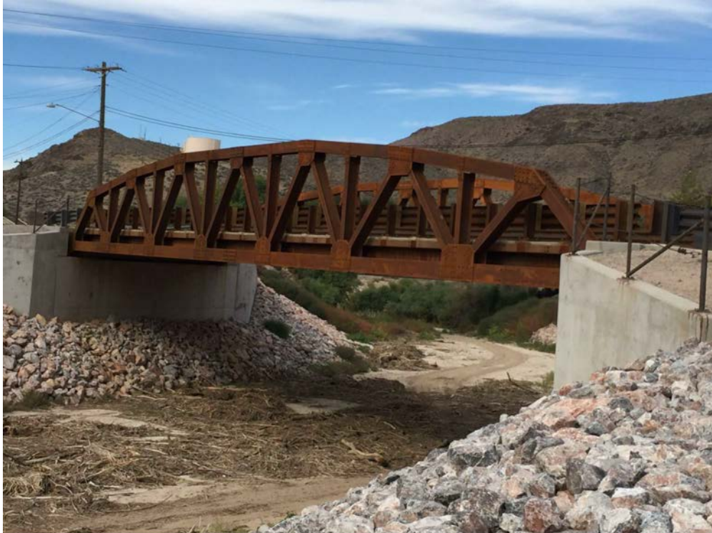
Photo 3. Clover Creek Crossing Structure – New Nevada DOT Bridge
