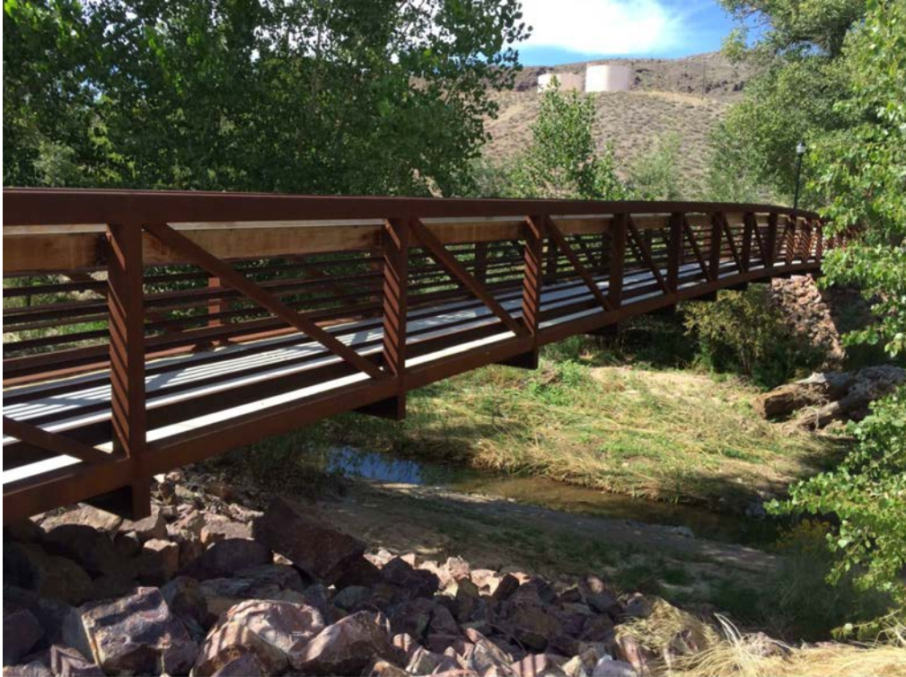
Photo 7. Meadow Valley Wash Crossing Structure – Elementary School Pedestrian Bridge
