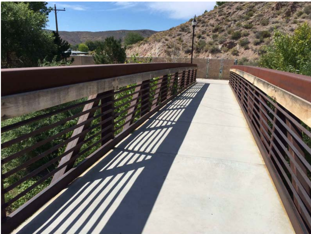
Photo 14. Meadow Valley Wash Crossing Structure – New Pedestrian Bridge 3
