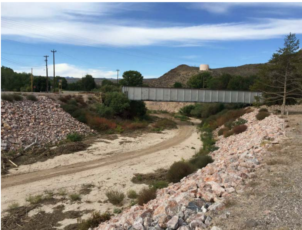
Photo 4. Clover Creek Crossing Structure – Abandoned Railroad Bridge
