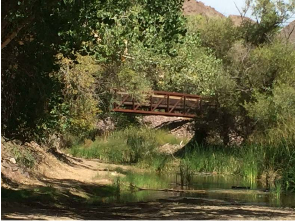
Photo 11. Meadow Valley Wash Crossing Structure – New Pedestrian Bridge 2
