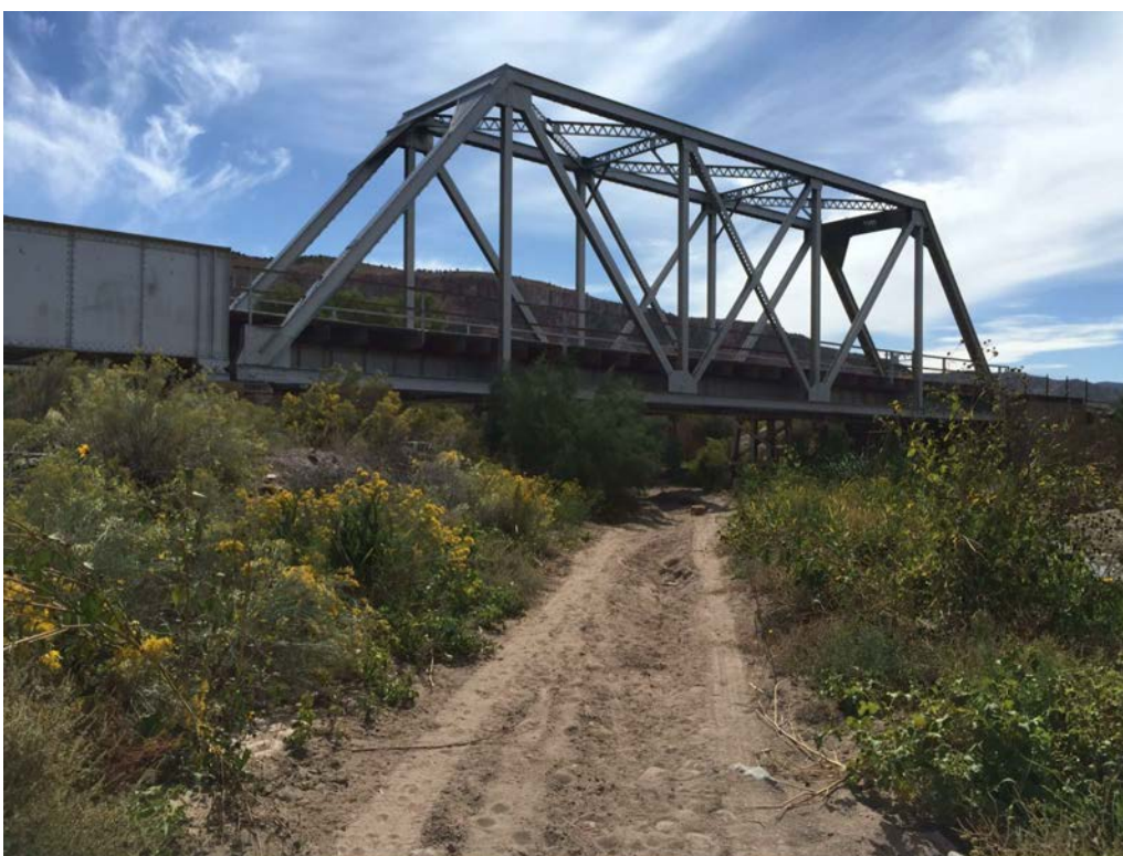
Photo 20. Meadow Valley Wash Crossing Structure – Union Pacific Railroad Bridge Southeast Caliente
