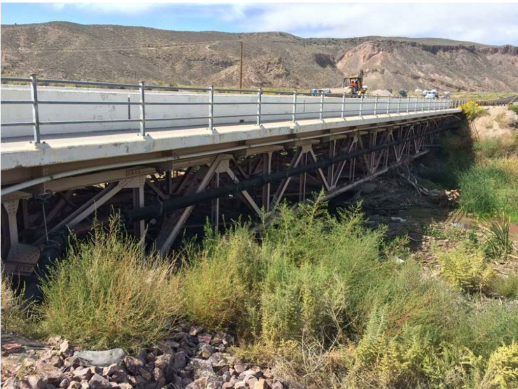
Photo 16. Meadow Valley Wash Crossing Structure – Southwest U.S. Highway 93 Bridge
