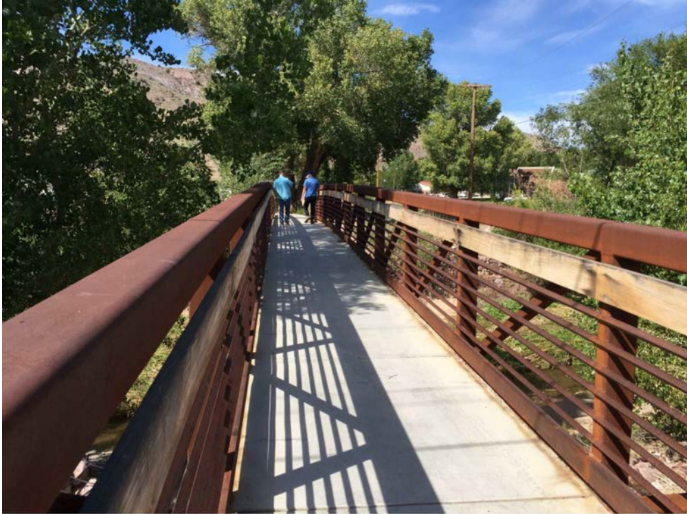
Photo 9. Meadow Valley Wash Crossing Structure – New Pedestrian Bridge 1
