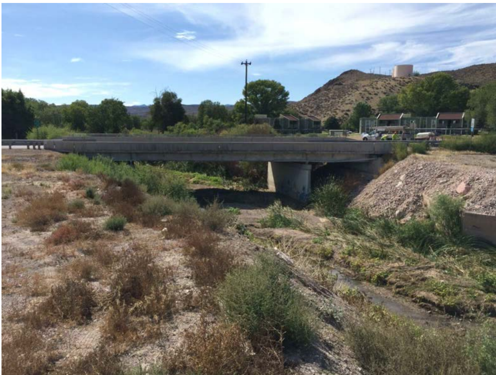
Photo 6. Meadow Valley Wash Crossing Structure – Northeast U.S. Highway 93 Bridge
