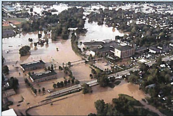
Figure 4-7. Floodwaters surround Columbus Regional Hospital in 2008
