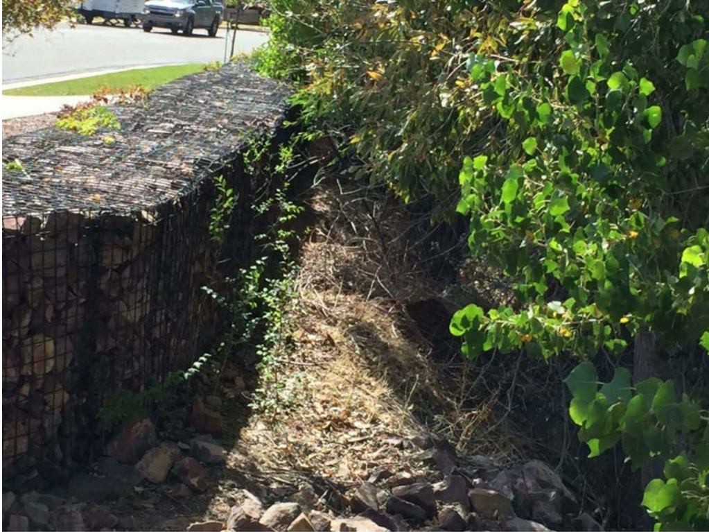
Photo 13. Meadow Valley Wash Linear Park – Gabion Wall
